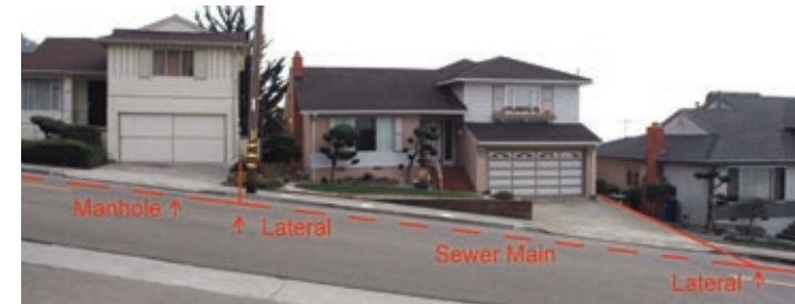
In this photo, the gray house is at risk. The pink house may be at risk if it has a floor drain in the garage. Most likely, the house on the left is not at risk.
