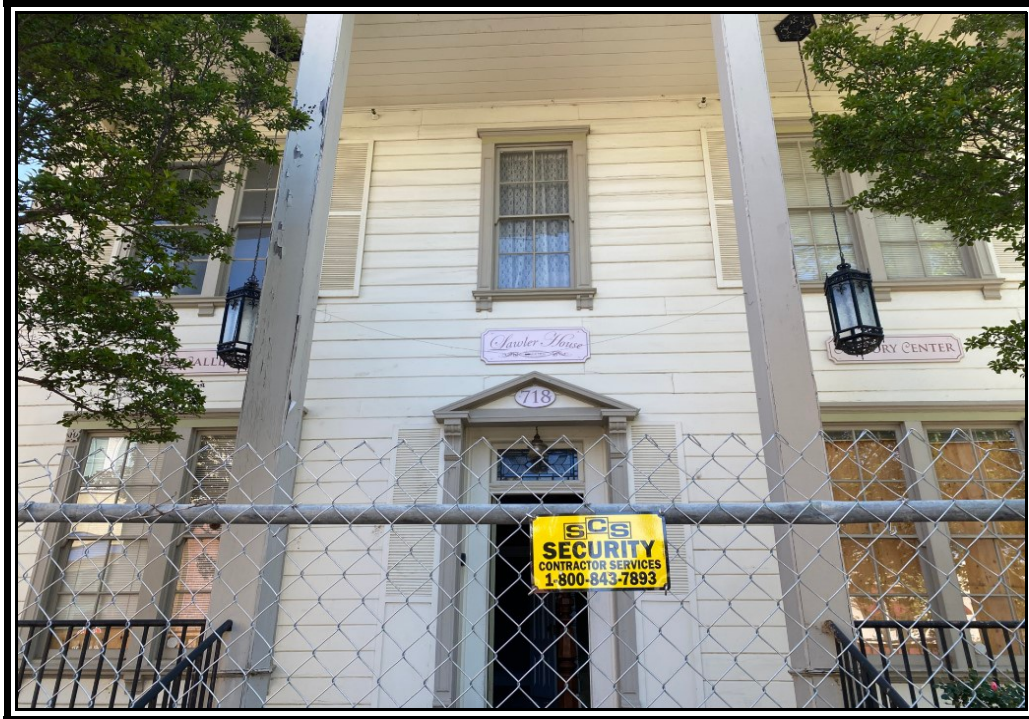
Front entrance to the subject property, currently fenced off. Damage is noted on the left pillar.
