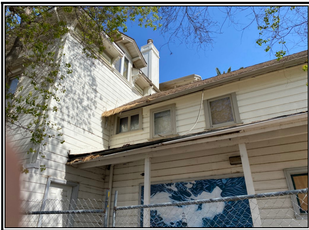
South side of the building which shows extensive roof and gutter damage. Note that both gutters in image are failing and show signs of vegetation growth that typically is associated with a build up of organic material over multiple years.
