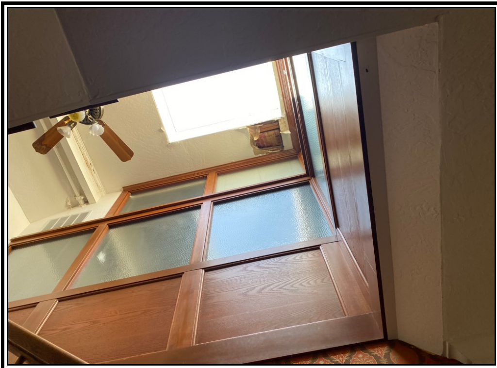
This is the view looking up the 2 nd floor stairwell that would access the 3 rd floor. We were not allowed access due to the excessive mold and unsafe conditions. Shown in the image is a large hole that has developed in the 3 rd floor ceiling due to excessive water damage.
