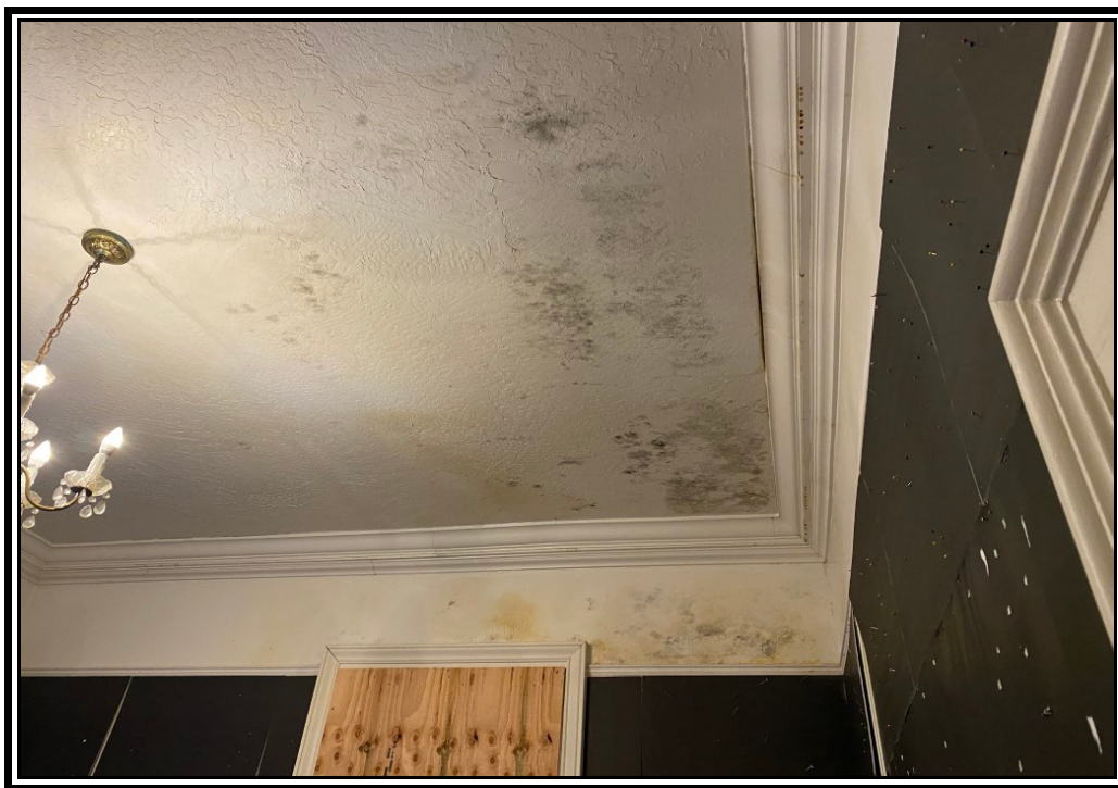
Extensive mold was found throughout the property as is evident on the roof and walls in this image.
