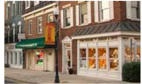
Upper floor facades should be composed of solid surfaces with punched openings for individual or sets of windows.
