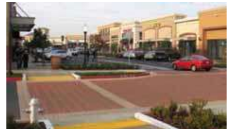
Color and different architectural treatments should be used to distinguish individual tenants in multitenant buildings.
