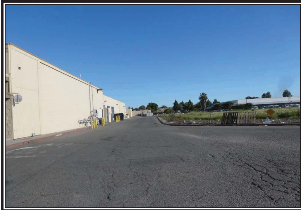
View north of the west end of the Subject. The subject is on the right, the rear of the post office is in the right background, and the rear of the Sunset Shopping Center is on the left
