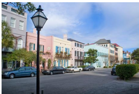
New storefronts along Main Street shall approximate the rectangular form, proportions, and character of adjacent buildings of historic interest.
