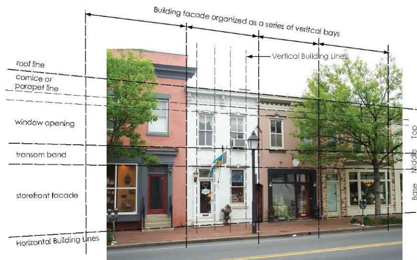
Storefronts along Main Street shall be designed as three bands that include a base, middle, and top.
