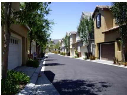
Garages shall be at the rear of the lot and accessed by an alley or motorcourt.
