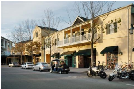
New larger buildings should use smaller-scaled elements that approximate the scale or form of adjacent residential development.
