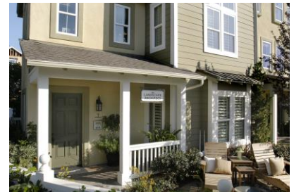
Exterior wall materials shall use traditional residential building materials, such as wood siding, stone, and brick.
