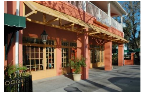
Traditional design features, such as wooden balconies, canopies, and porches shall be used.
