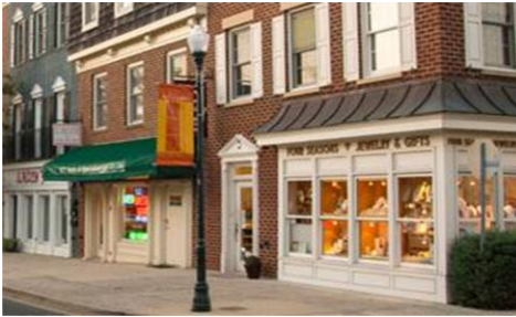
Upper floor facades shall be composed of solid surfaces with punched openings for individual or sets of windows.
