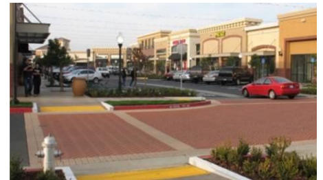
Color and different architectural treatments shall be used to distinguish individual tenants in multitenant buildings.
