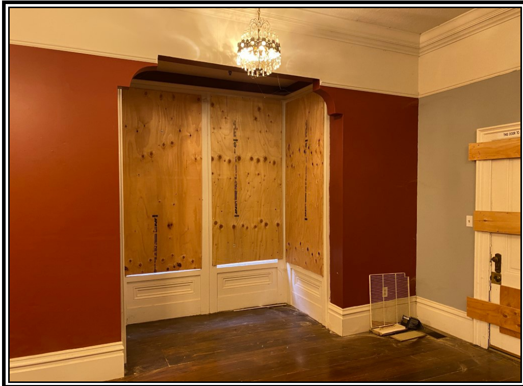
Boarded up windows on the ground floor due to repeated break-ins.
