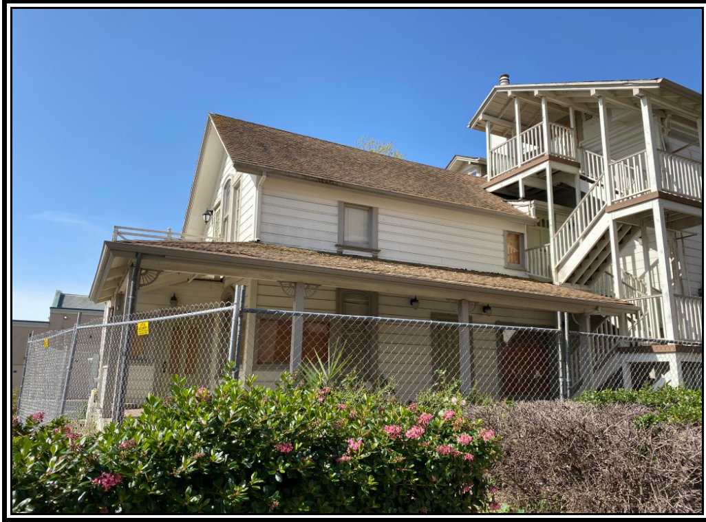
Northeast corner of the subject building.
