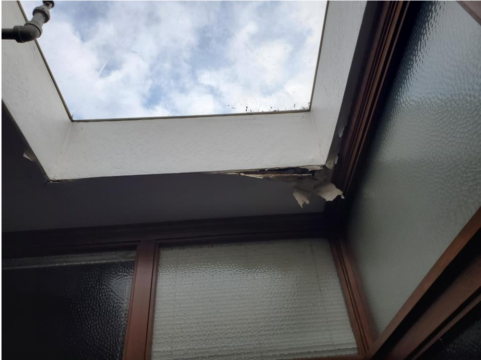
Leaking skylight with damaged ceiling
