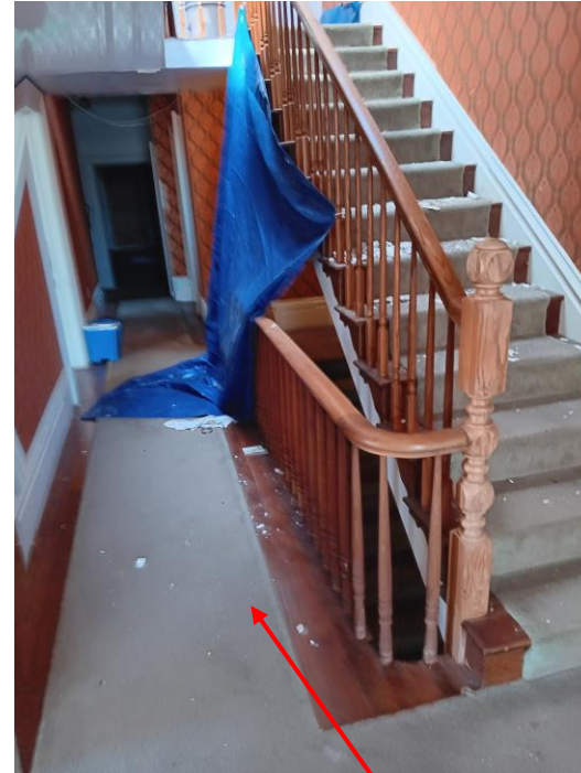
Extensive water leaks & damage in hallway and stairs to the 3 rd Floor from skylight and roof.
