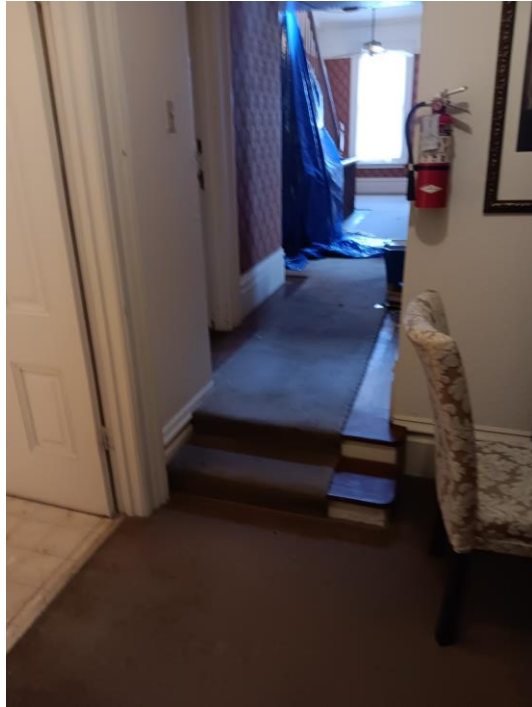
Landing for exterior stairs
