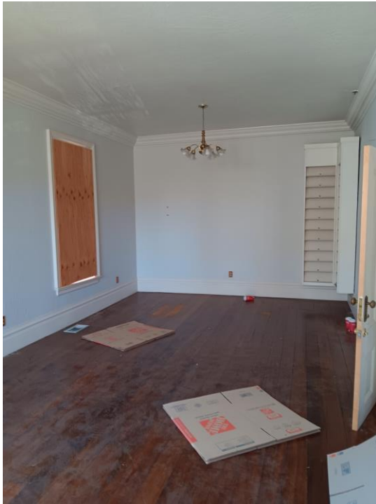
Office 1 (front of building, left side)
