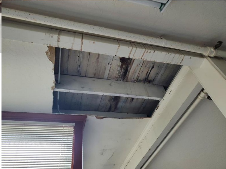
Roof beam water damage
