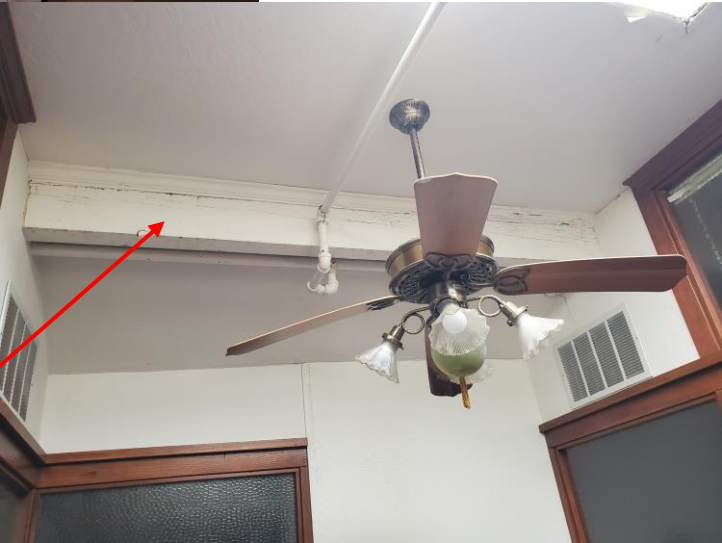
Leaking skylight with damaged ceiling
